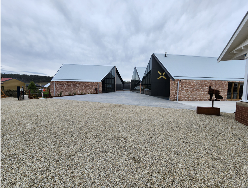
New distillery showing the new concrete pavement. Photo by Hamid Saeidi
