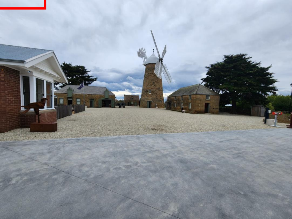
Photo 2: View of the Heritage listed buildings site from the east looking in a western direction. The edge of the hardstand is contained within CT 240022/1 and does not encroach on the adjacent Crown land (source: Callington Pty Ltd)
