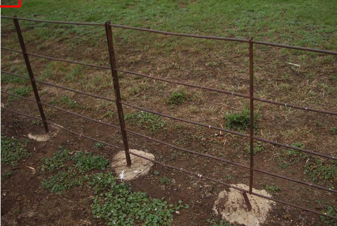
Iron 'estate' fencing to be used. This is a colonial example from Woolmers Estate which will be replicated for this project.
