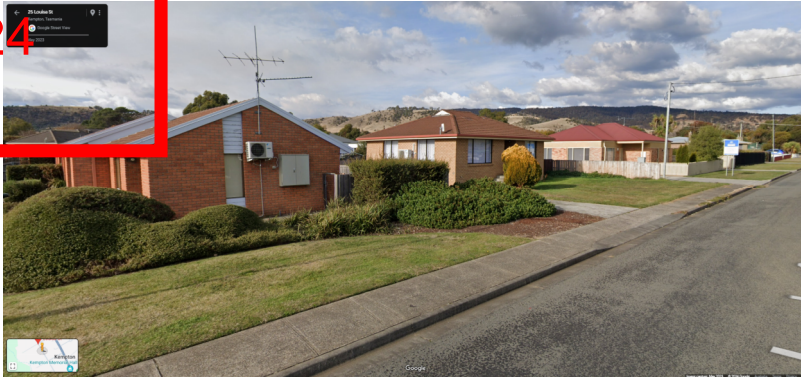
Fig 1 Residential properties on Louisa Street clad in brick veneer and lightweight cladding accents
