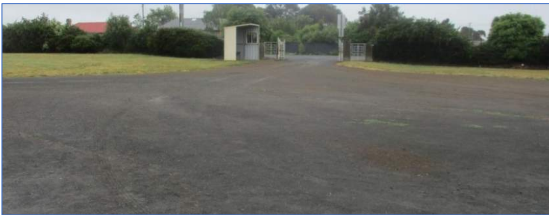
Photograph 5.4A – Existing internal driveway adjacent to High Street
