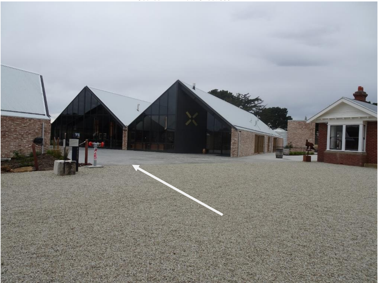
Image.5. New distillery buildings at 99 High Street in the centre and left of the image which are located internally within the subject site. The adjacent red brick miller's Cottage can be seen on the right. Gravelled landscaping in the foreground is located within the Callington Mill site at 6 Mill Lane. The concrete works have been arrowed.
