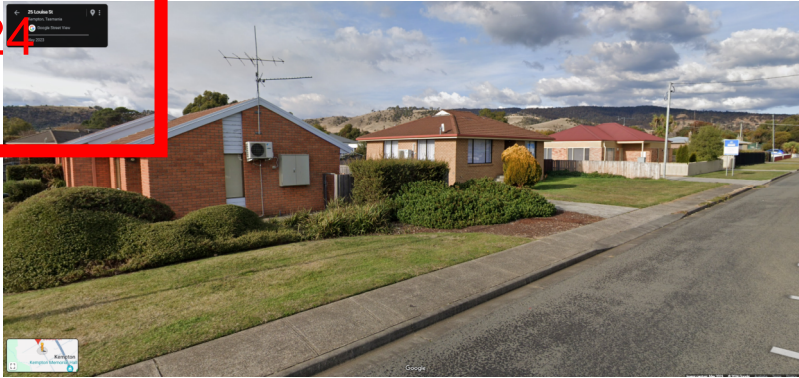
Fig 1 Residential properties on Louisa Street clad in brick veneer and lightweight cladding accents
