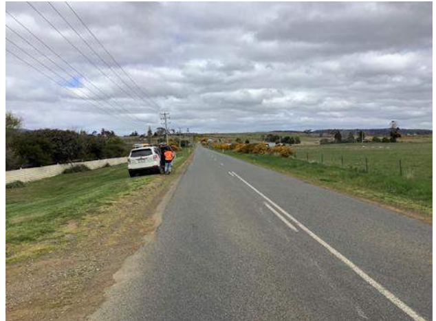
Figure 7: Tunnack Road - facing south
