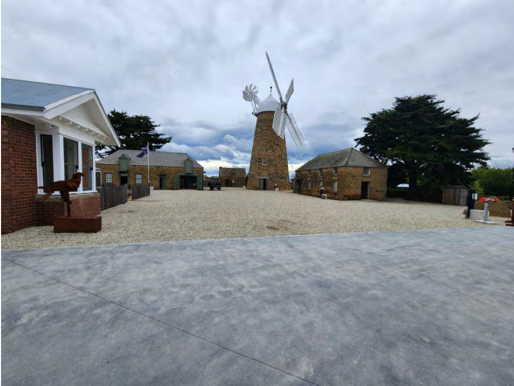
Photo 2: View of the Heritage listed buildings site from the east looking in a western direction. The edge of the hardstand is contained within CT 240022/1 and does not encroach on the adjacent Crown land (source: Callington Pty Ltd)
