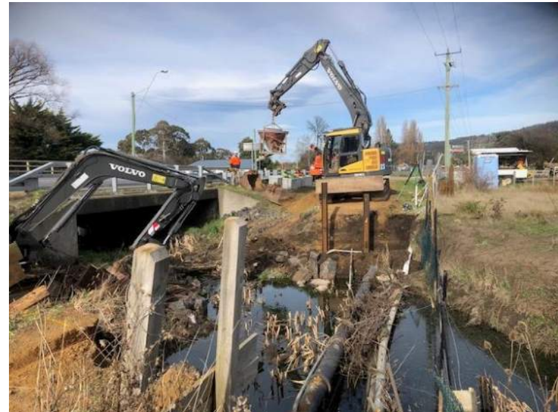
New 2.5m wide Footbridge under construction
