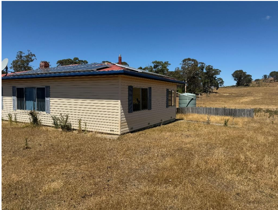
Figure 12 – Existing managed land and dwelling within Lot 1, (view facing SE)
