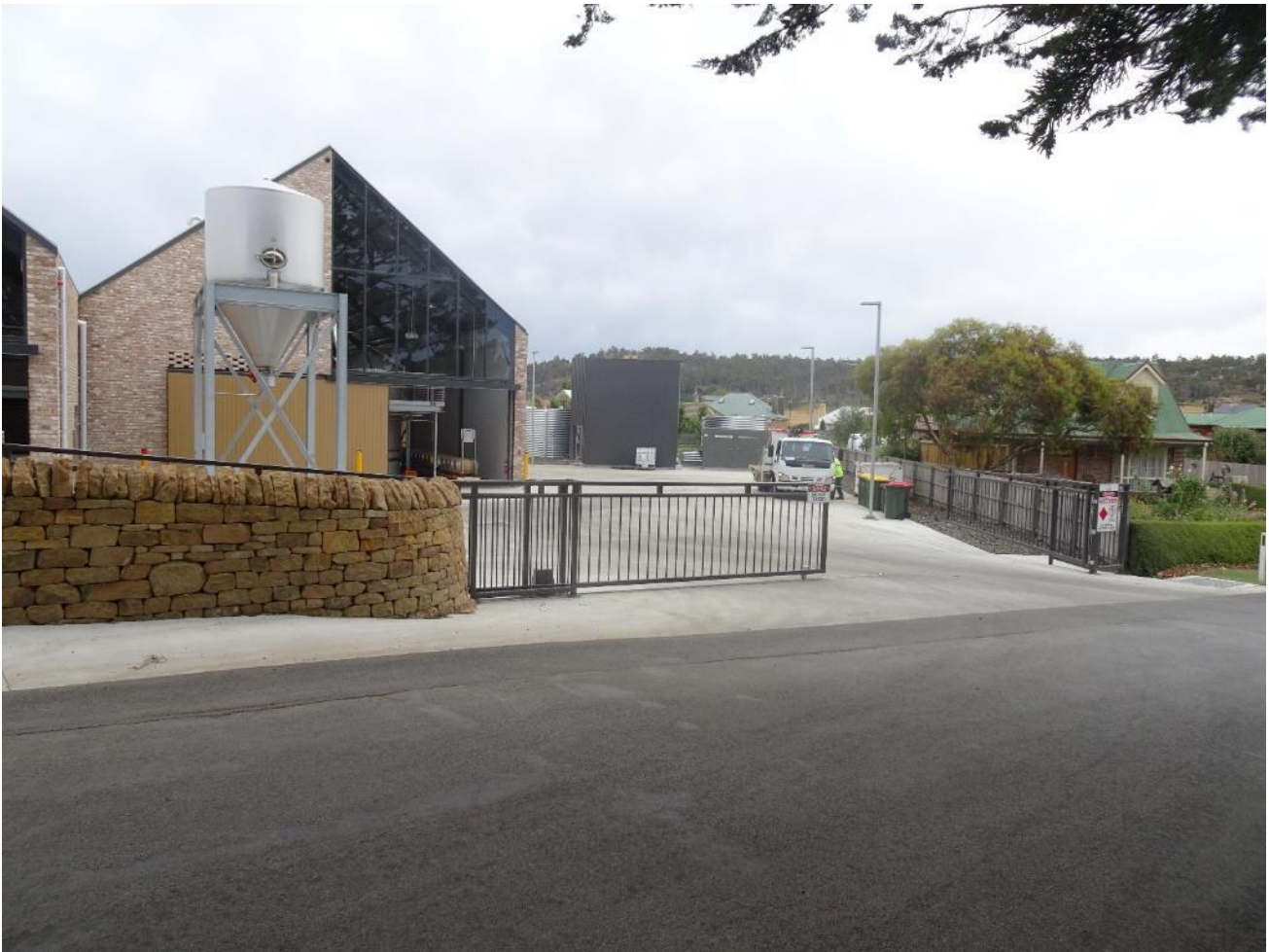
Image.8. New distillery buildings at 99 High Street fronting the Esplanade. The grey concrete hard landscaping that is the subject of this application for an approval under the Southern Midlands LPS and Tasmanian Planning Scheme (State Planning Provisions) can be clearly seen both within the service area of the subject site and also in the crossover and road reservation area.
